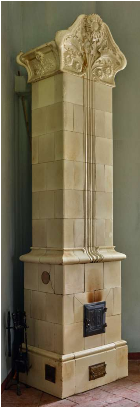
Fig 6: The reconditioned stove from Făgăraș with its jugendstil sunflower. The other stoves are newly made
