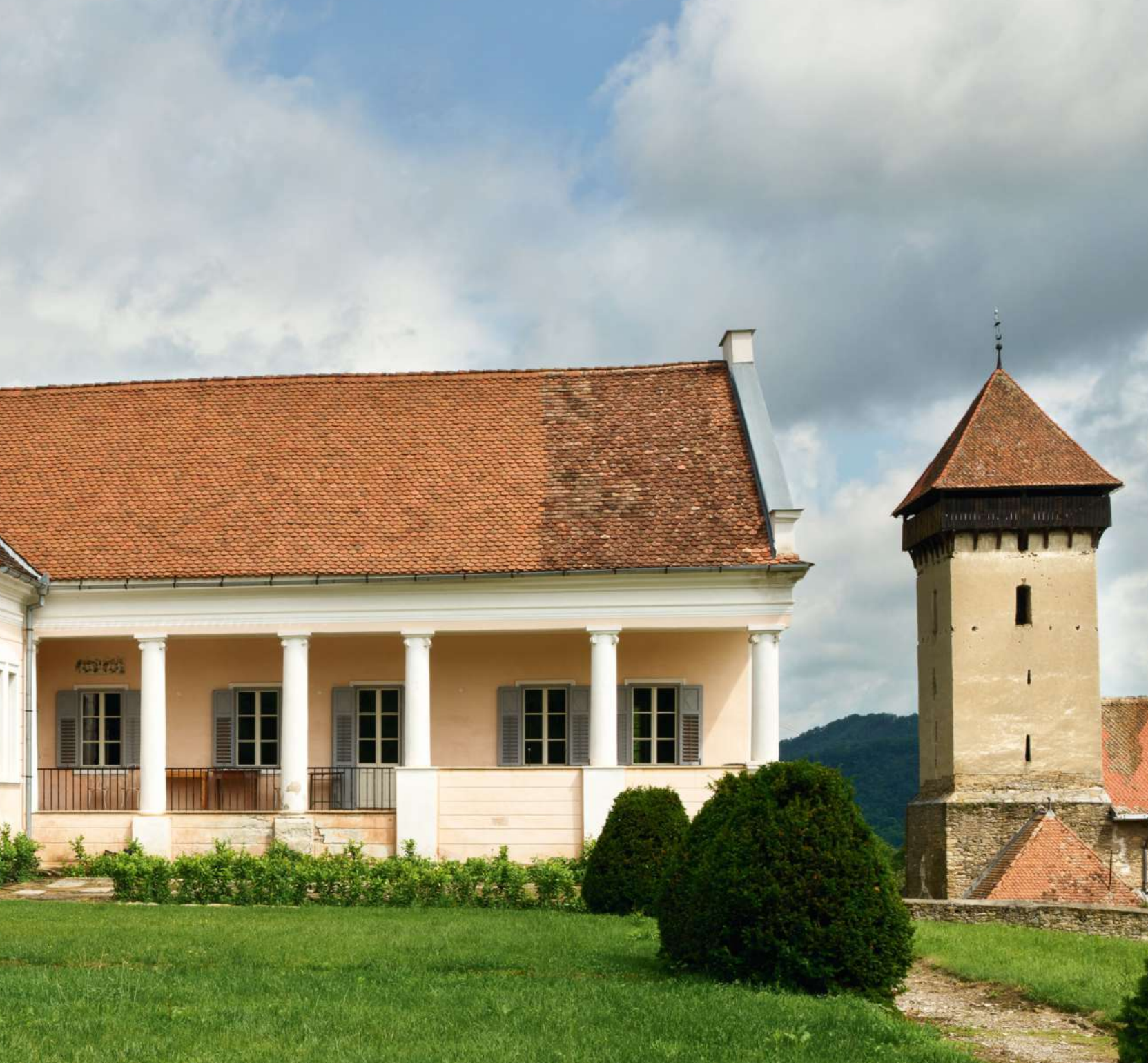
Fig 1: The loggia and porch impose order on the asymmetric garden frontage of Apafi Manor, named for the princely family who built it. Much of the building to the left of the porch has been reconstructed. The parish-church tower is visible to the right
